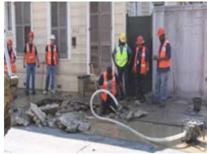
A group of workers repairing a water supply system
