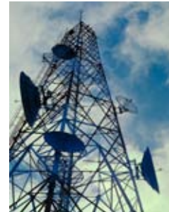
Ac ommunication tower
