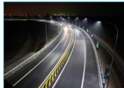
Electricity for streets
